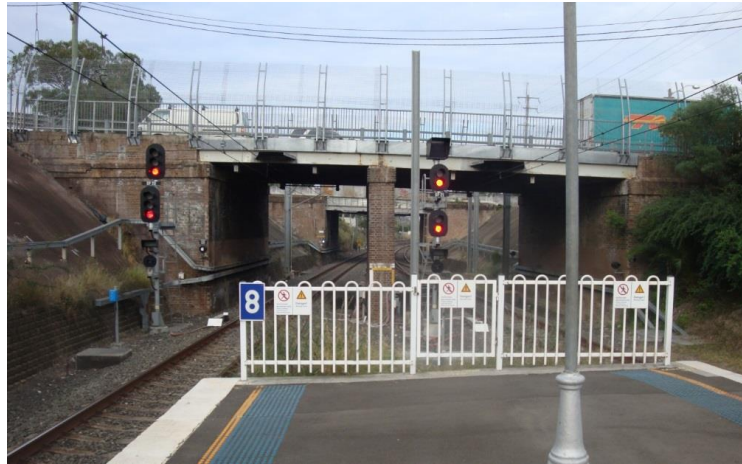
Figure 1. Existing Amy Street overbridge as viewed from Regents Park Station
