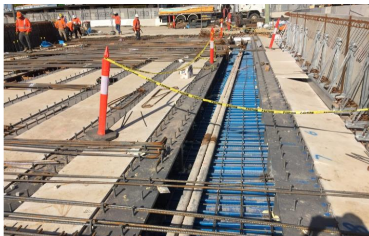
Figure 13. Work on the deck slab commenced upon completion of girder installation
