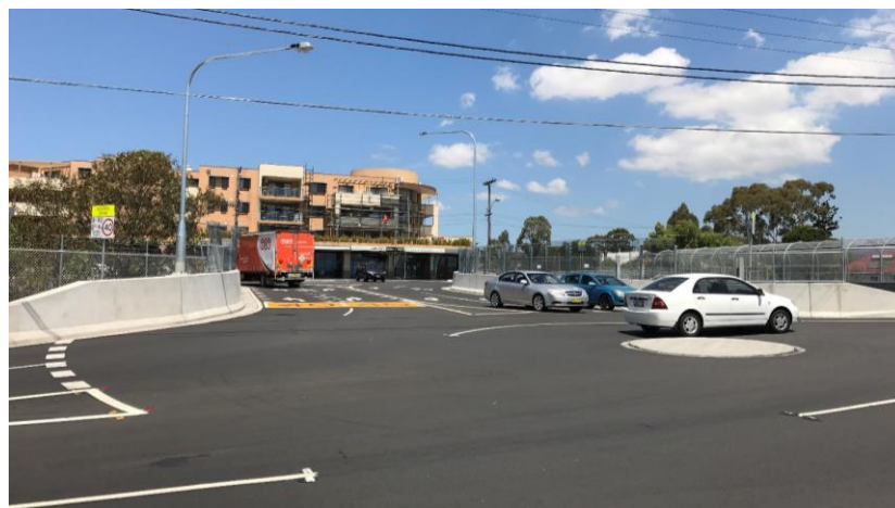
Figure 16 - New overbridge today as viewed from road level
