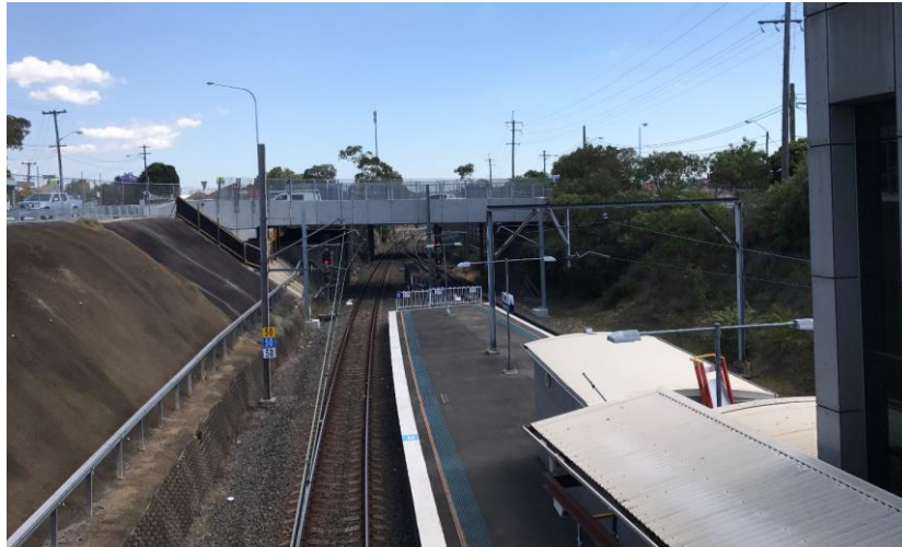
Figure 15 – New overbridge today as viewed from Regents Park Station
