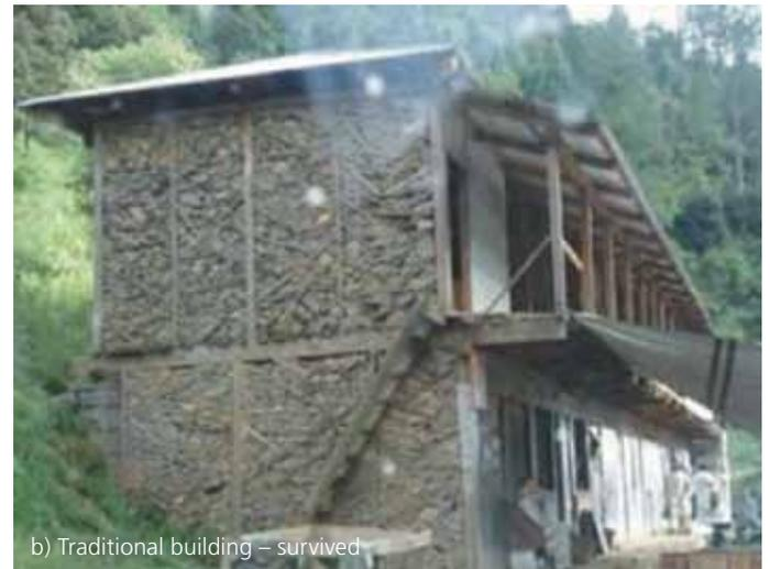
Figure 3: Comparing performance of modern and traditional construction in the 2005 Kashmir earthquake
