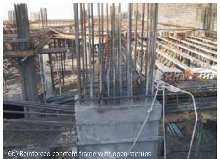
6b) Reinforced concrete frame with open stirrups
