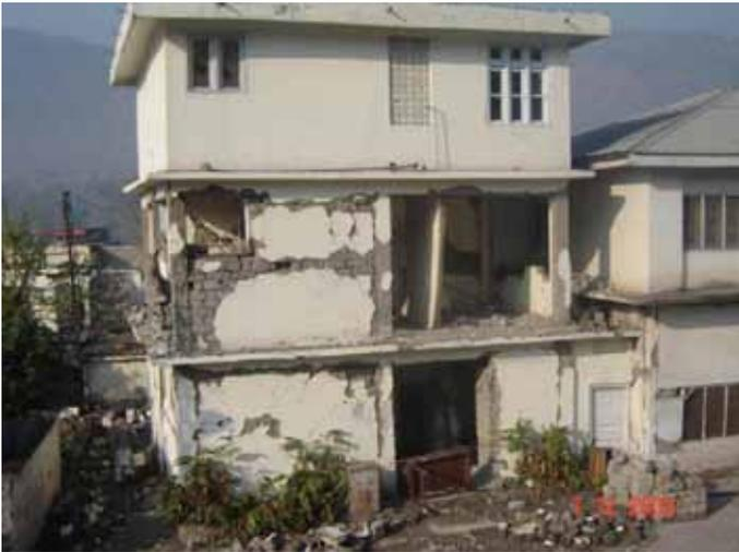
Figure 5. A typical reinforced concrete frame building with concrete block infill wall.
