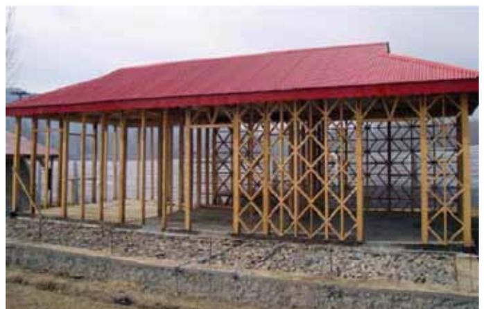
b) Implementing remedial measure for seismic safety.
