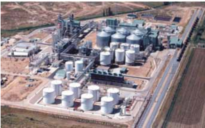
Figure 3: Abengoa, Castilla, Spain.
