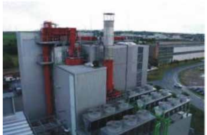
Figure 6: Choren, Freiburg, Germany
