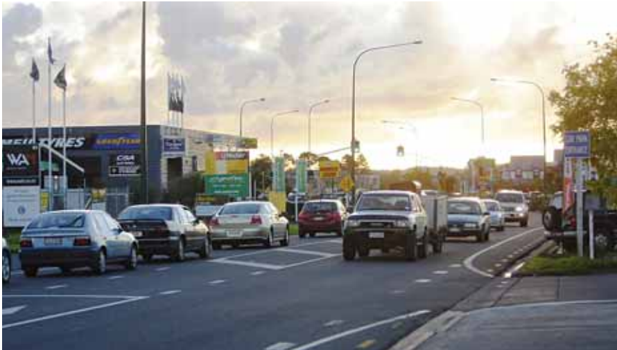
▲ SH16 – existing situation: The strategy seeks to improve the strategic transport network while also addressing safety concerns and enhancing amenity
