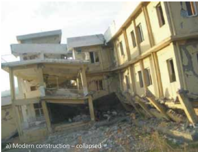
Figure 3: Comparing performance of modern and traditional construction in the 2005 Kashmir earthquake
