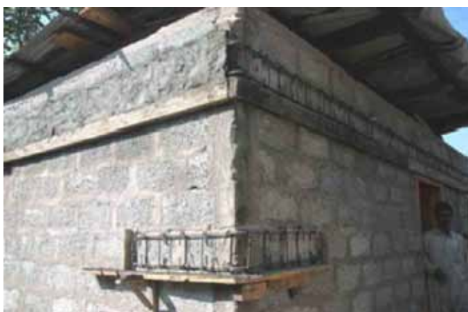
a) A Dhajji under construction.
