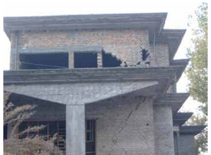
Figure 4. A typical brick masonry building.
