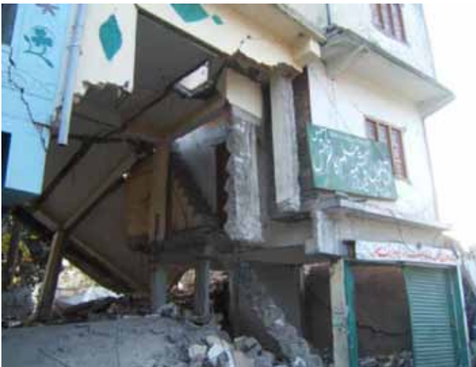
b) Reinforced concrete frame building on top of masonry building.
