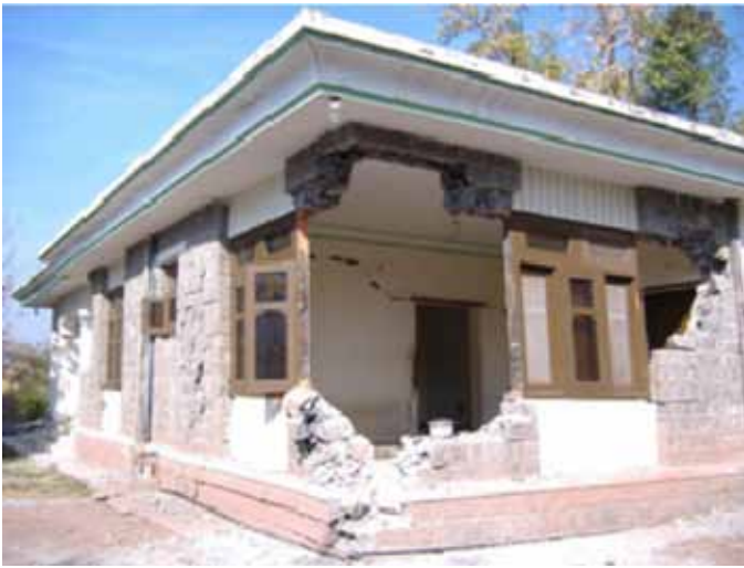
a) A modern stone masonry building
