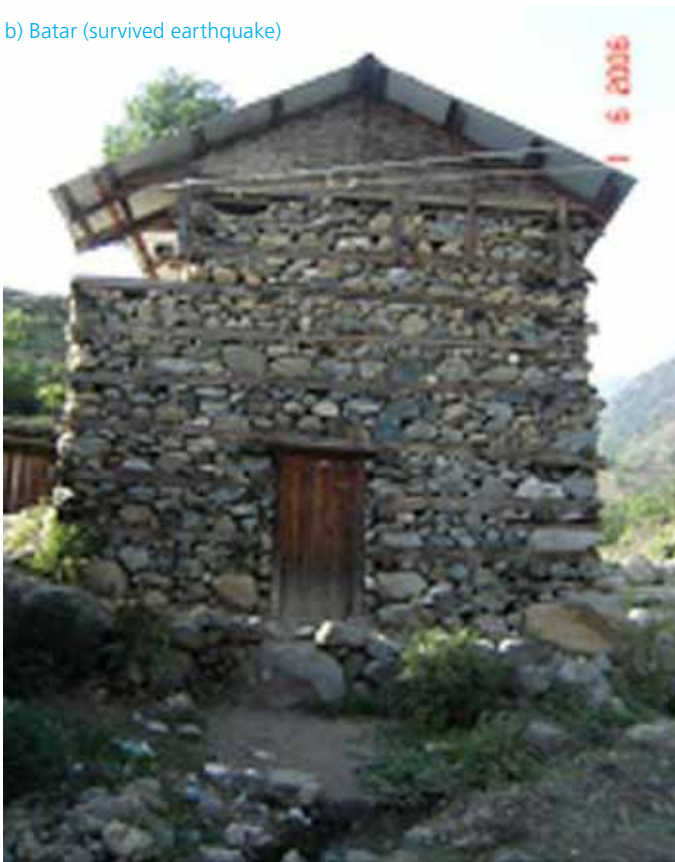
Figure 3. Excellent performance of traditional stone masonry buildings
