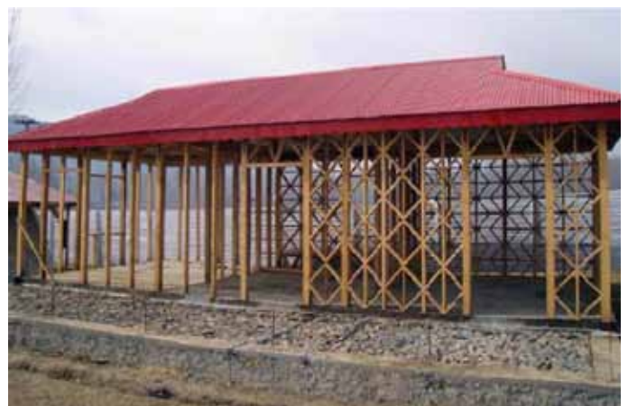
b) Implementing remedial measure for seismic safety.
